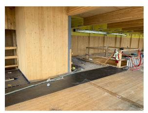
**Step 3:** Using **GenieMat Tape ST3**, tape all the seams to seal the **GenieMat**<sup>®</sup> **FF** system when a concrete topping is to be applied.
